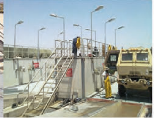
Wash rack systems:
